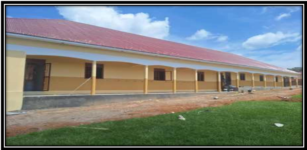
One of the new dormitory blocks at Hopeland High school Naija.
